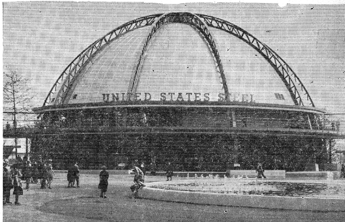
THE INSIDE OUT BUILDING . . . the United States Steel Corporation building is just that for the structural steel girders have been placed on the exterior of the edifice to emphasize the importance of steel in construction.
