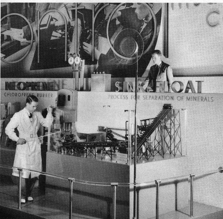
Here is demonstrated the operation of the "Sink-and-Float" process by means of a small plant model that separates pieces of coal from slate.
