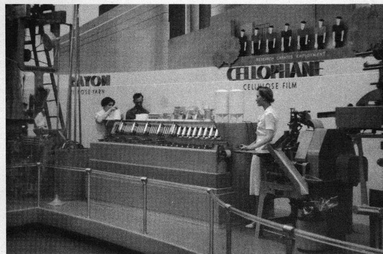
Here, the process of manufacturing "Cellophane" cellulose film from the raw material to the finished sheet is visualized. At the right is a candy-wrapping machine which turns out individually-wrapped pieces.
